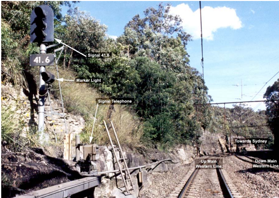
Figure 11 - View of Signal 41.6 showing position of marker light and signal telephone
