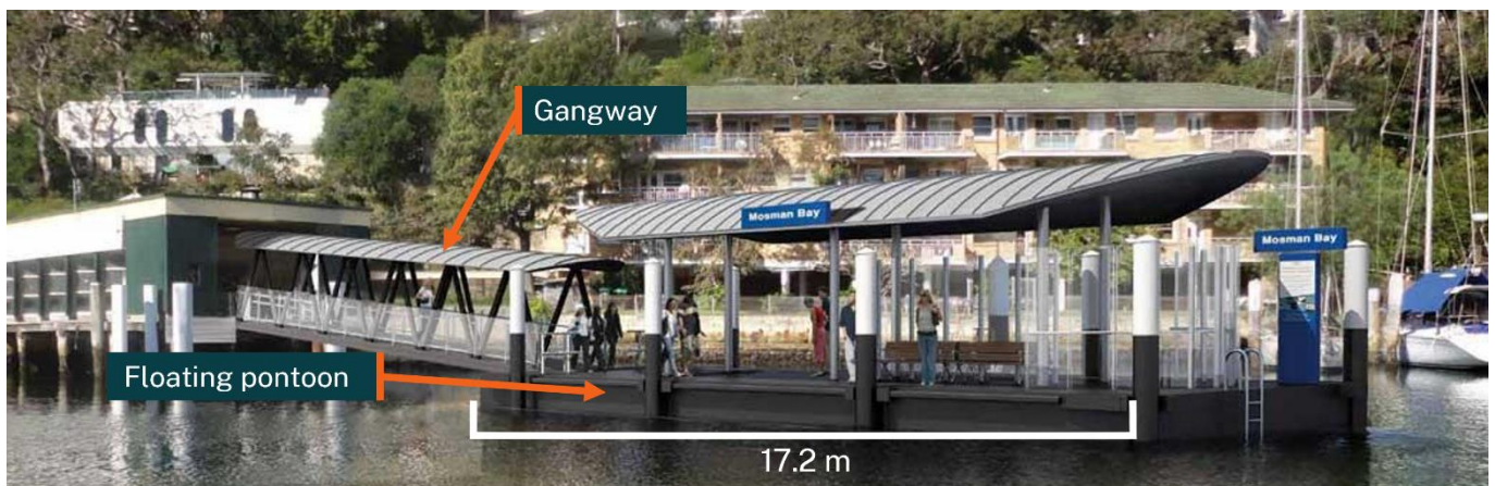
Figure 35: Mosman Bay wharf and gangway – Floating pontoon structure
