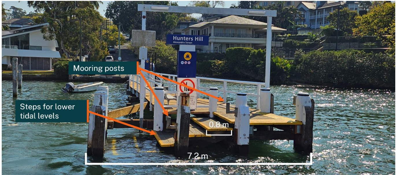
Figure 36: Hunters Hill Wharf – fixed structure
