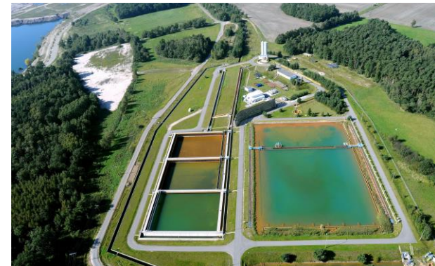
Water treatment plants
