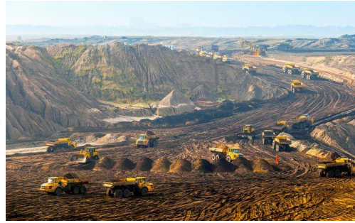
Preparation – earth moving
