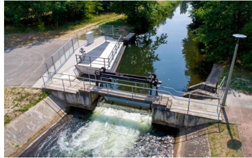
Flooding - river water
