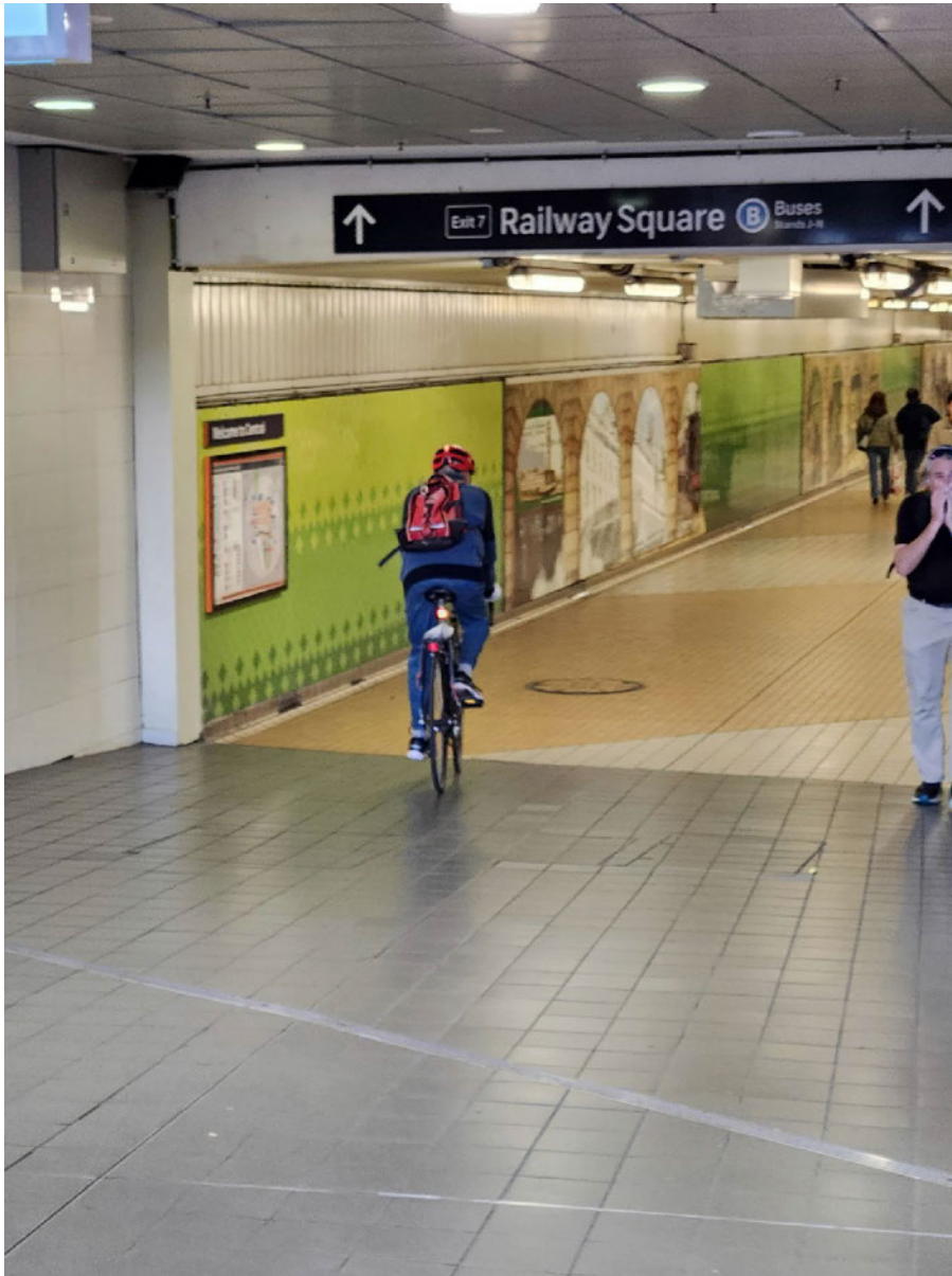
Fig. 16: Devonshire Street pedestrian tunnel
