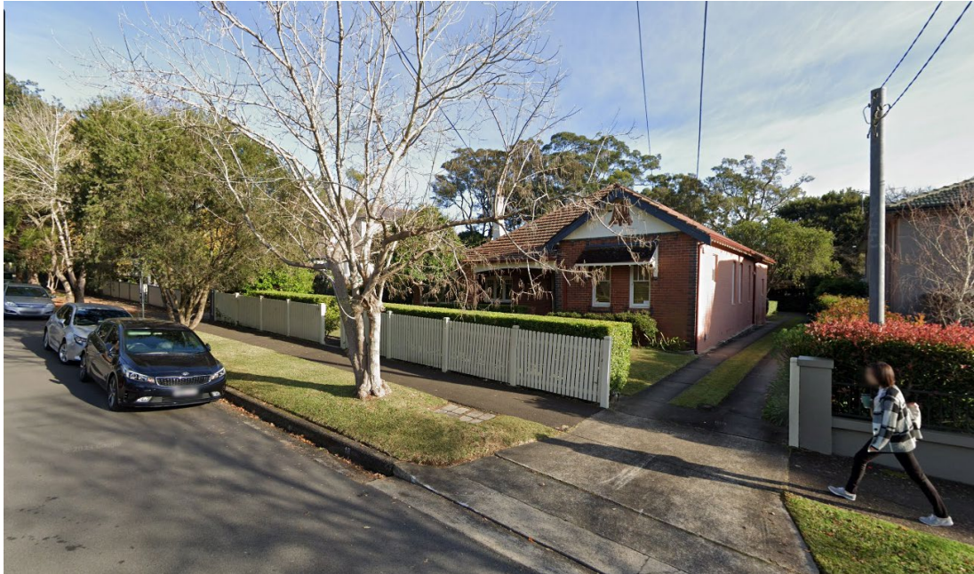
Above: Clanville conservation area, Roseville Avenue, proposed for 6-7 storey apartments
