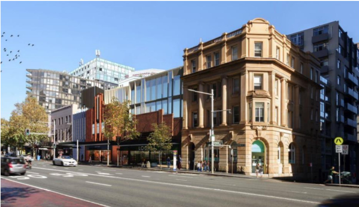
Figure 6. Alterations and vertical additions to 21-35 Oxford Street, Darlinghurst for office, cultural and creative uses
