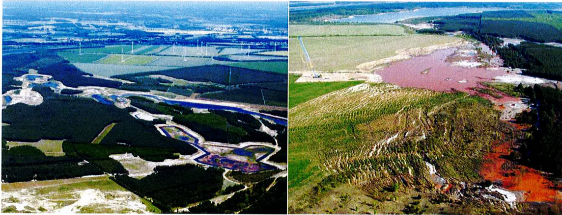
land subsidence in the former Seese-West mine area (left 2010, right 2011 after subsidence) Source: LMBV
