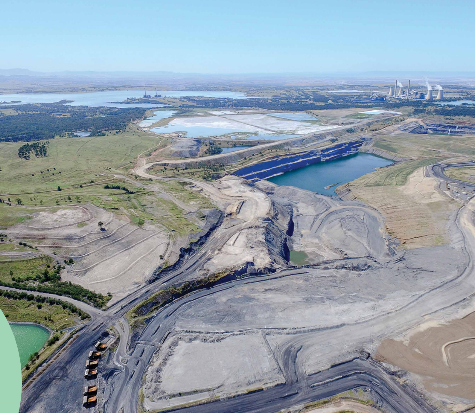
ABOVE: Drayton coal mine, coal ash dams, and Bayswater power station in the background.
