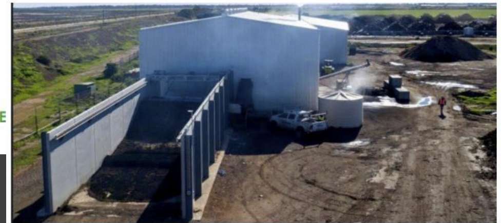
FIGURE 8 JEFFRIES PYROCAL SYSTEM OPERATING IN 2022
