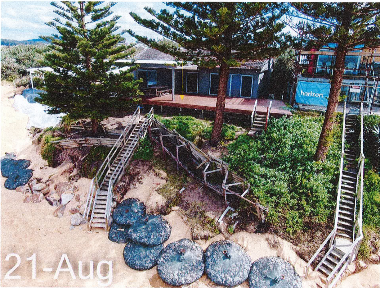
Figure 4: View of rock bags at site (at arrow) on 21 August 2020
