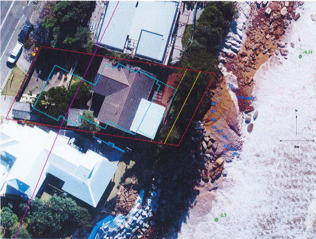
Figure 6: Aerial view of site (surveyed boundary in red) on 20 July 2020, with AHD levels of exposed clay/weathered rock in blue, Coastal Building Line in magenta, MHL (2022) seawall alignment in solid yellow (3m landward dashed yellow), Coastal & Marine Geosciences (1997) bedrock levels in green, and proposed Level 1 outline in cyan (dwelling solid and deck dashed)
