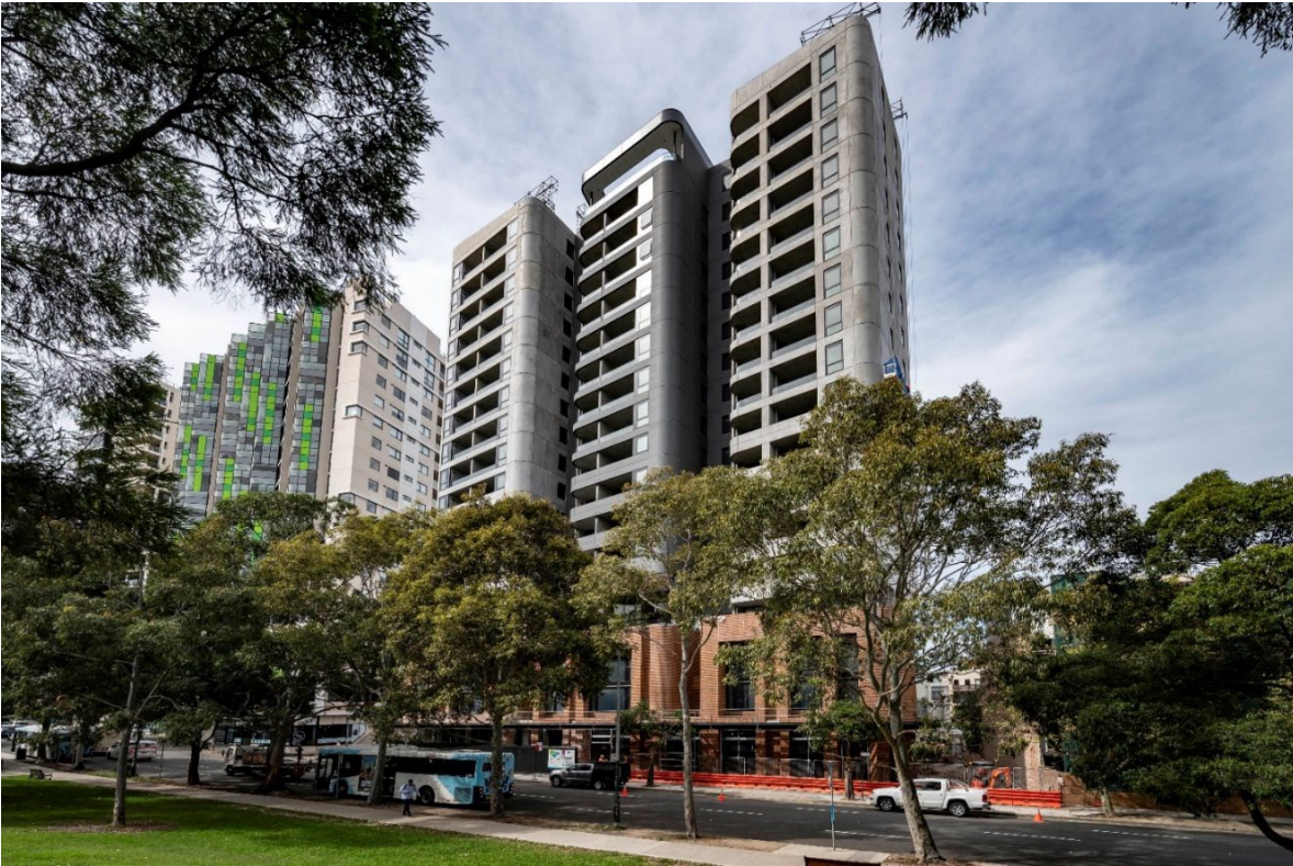
18 storey, 165 unit, Affordable Housing, 11 Gibbons Street, Redfern 2021. St George Community Housing, built on former City of Sydney Depot site.
