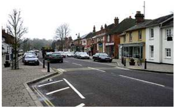
This road narrowing in Britain improves the visibility of pedestrians to drivers and reduces the time pedestrians need to cross the road. Note the bollards to make the buildout more visible to drivers, and the curb ramps with tactile warning tiles for visually impaired pedestrians.
