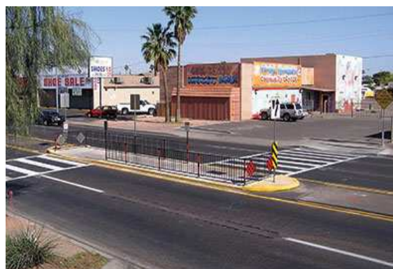
Two-stage crosswalks like this one in Phoenix are the result of pedestrian safety initiatives taken by the city with technical support from FHWA. This countermeasure is helping to reduce pedestrian-vehicle crashes in Arizona. Note the fence to help protect pedestrians as they cross the street.
