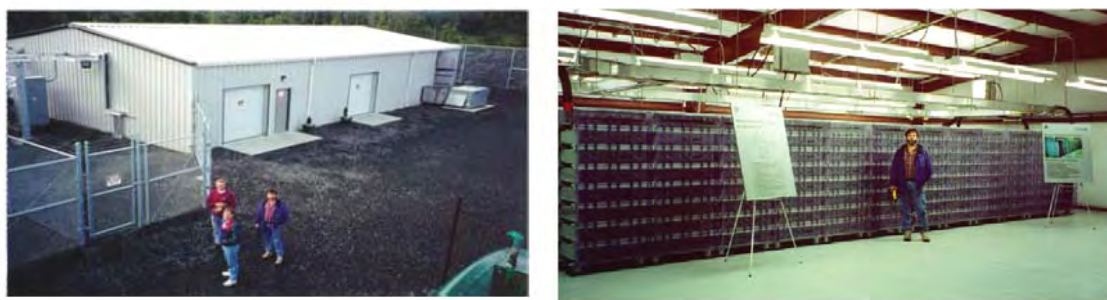
Figure 4-7 1-MW/1.5-MWh Lead-Acid System at Metlakalta, Alaska
