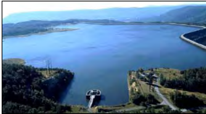
Figure 4-3 Manmade Upper Reservoir of TVA's Raccoon Mountain Pumped Hydro Plant. Operational in 1979, the facility can generate 1620 MW for up to 22 hours.
