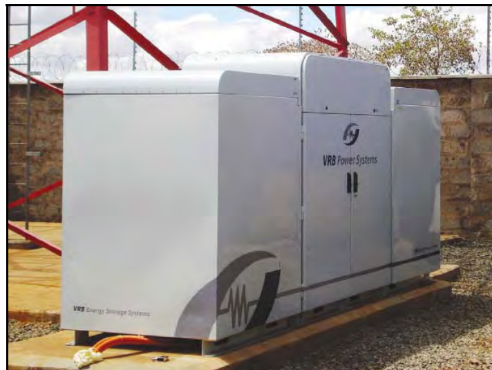
Figure 4-12 Prudent Energy 5-kW/30-kWh VRB-ESS installed at Kitangi, Kenya works alongside a diesel generator to comprise a hybrid power system at an off-grid site.
