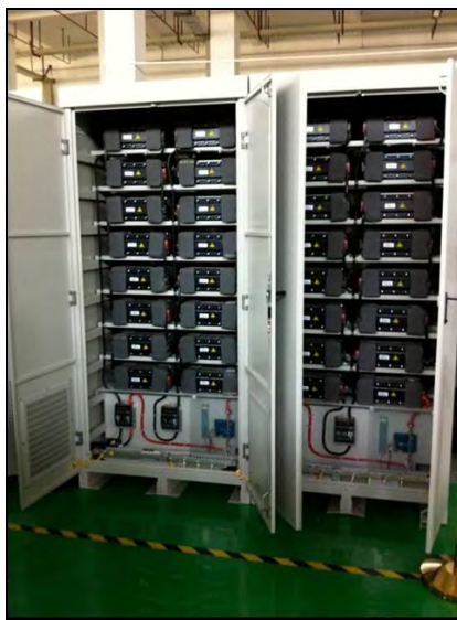
Figure ES-8 A 50-kWh BYD Li-ion Battery System Planned to be Tested at EPRI's Knoxville, Tenn. Smart Grid Laboratory in 2011.
